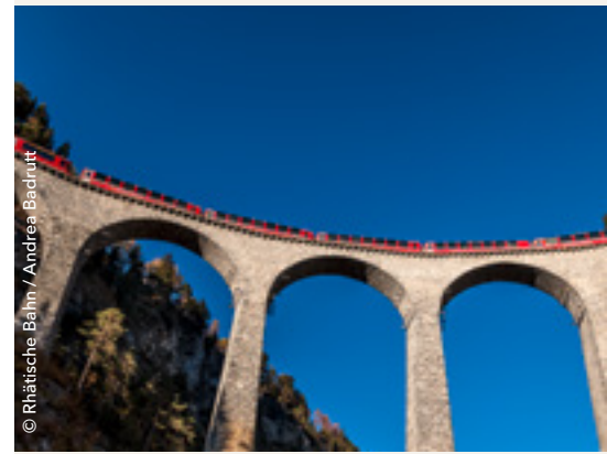
Bernina Express, Landwasser viaduct
